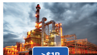
Gas Processing Facilities
