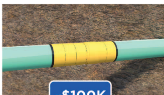
In Situ Pipeline Repair
